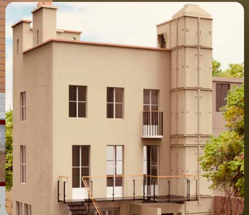
East Village Carriage House - Upgraded with a Lift to allow aging residents to live in a 3 story.
